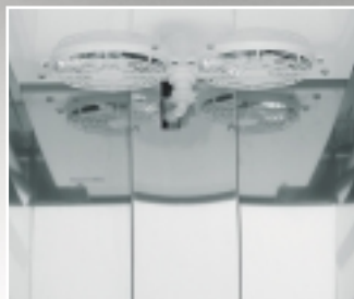
Evaporator above in 1-part version
